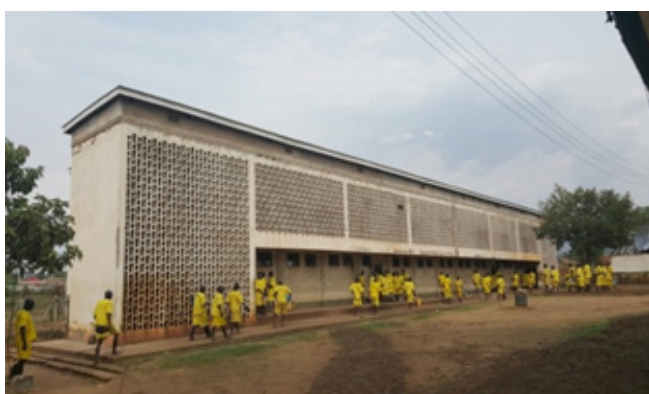
Re-roofed Prisoners' wards at Mbale Prison
