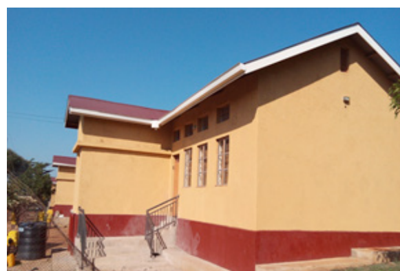
Completed renovation of Prisoners wards at Tororo
