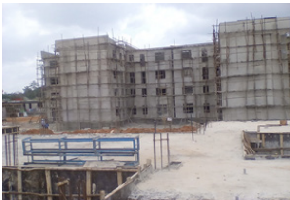
One of the blocks near completion at Naguru UPF staff housing project
