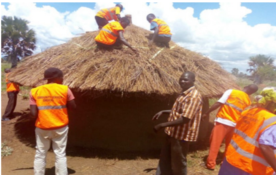
Offenders roofing a teacher's house at Kijo P/S, Gulu
